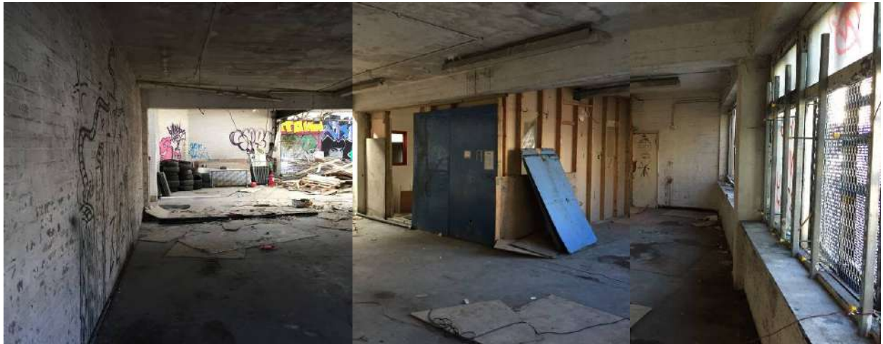
Internal view of Northern Building
