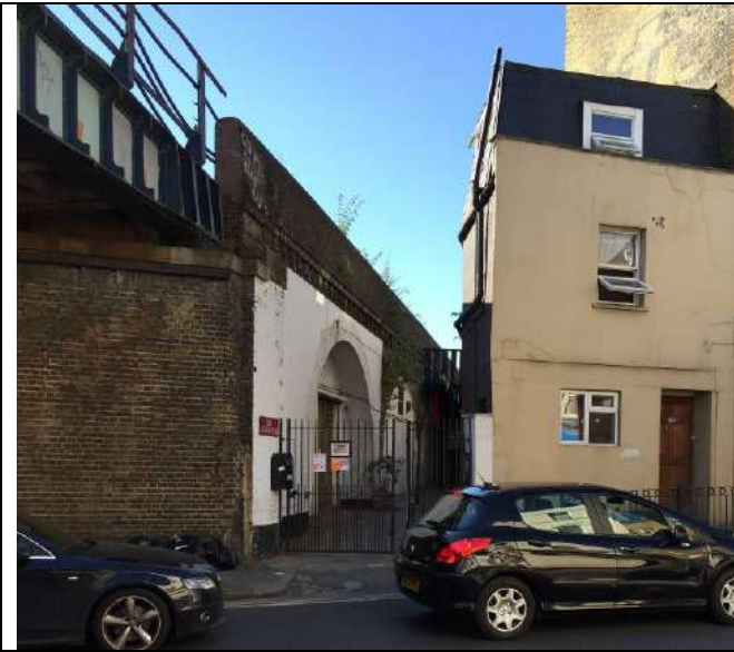
View Looking South from Coldharbour Lane of railway east of site
