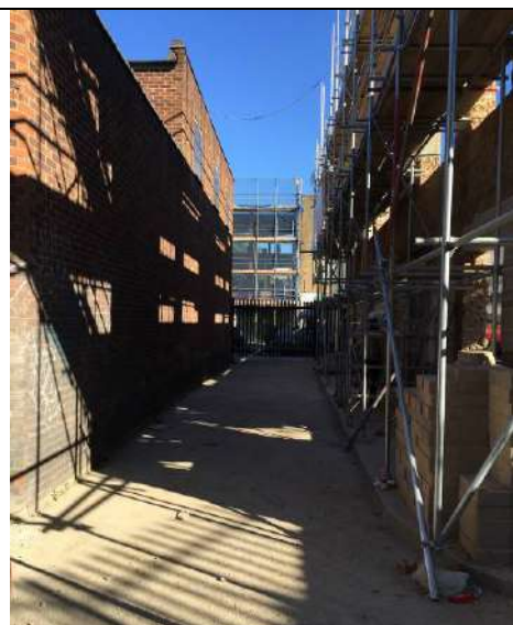
View of site Access Looking Northwest
