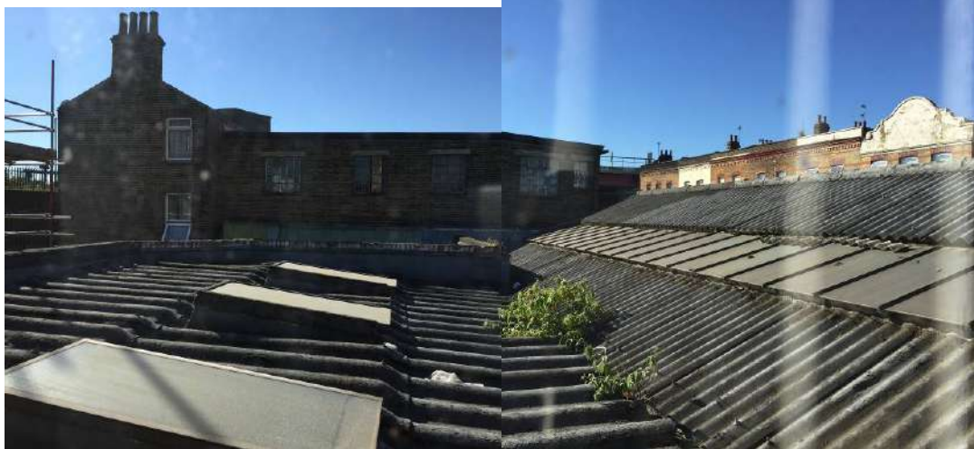
Roofscape Looking Southeast from first floor
