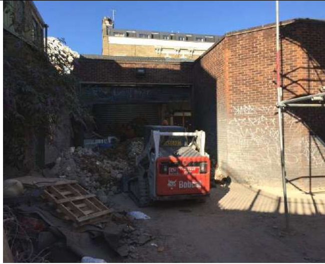
View Looking Southwest from Turning Head towards Building
