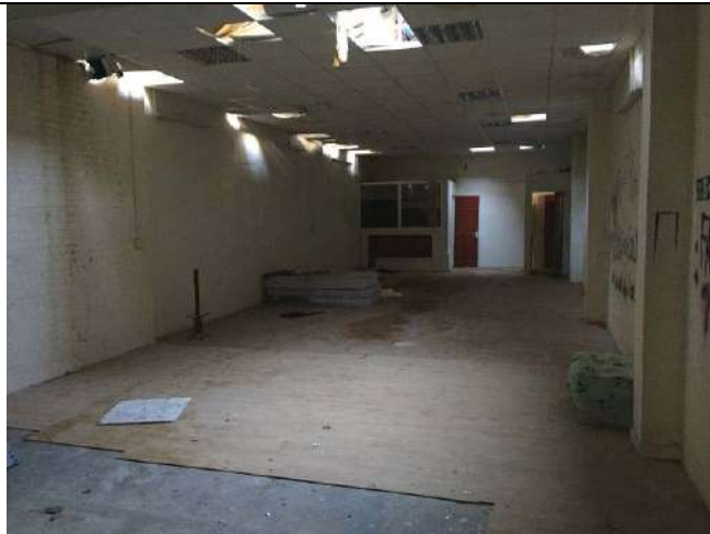
Internal view of Southern Building
