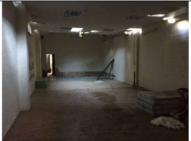
Internal view of Southern Building
