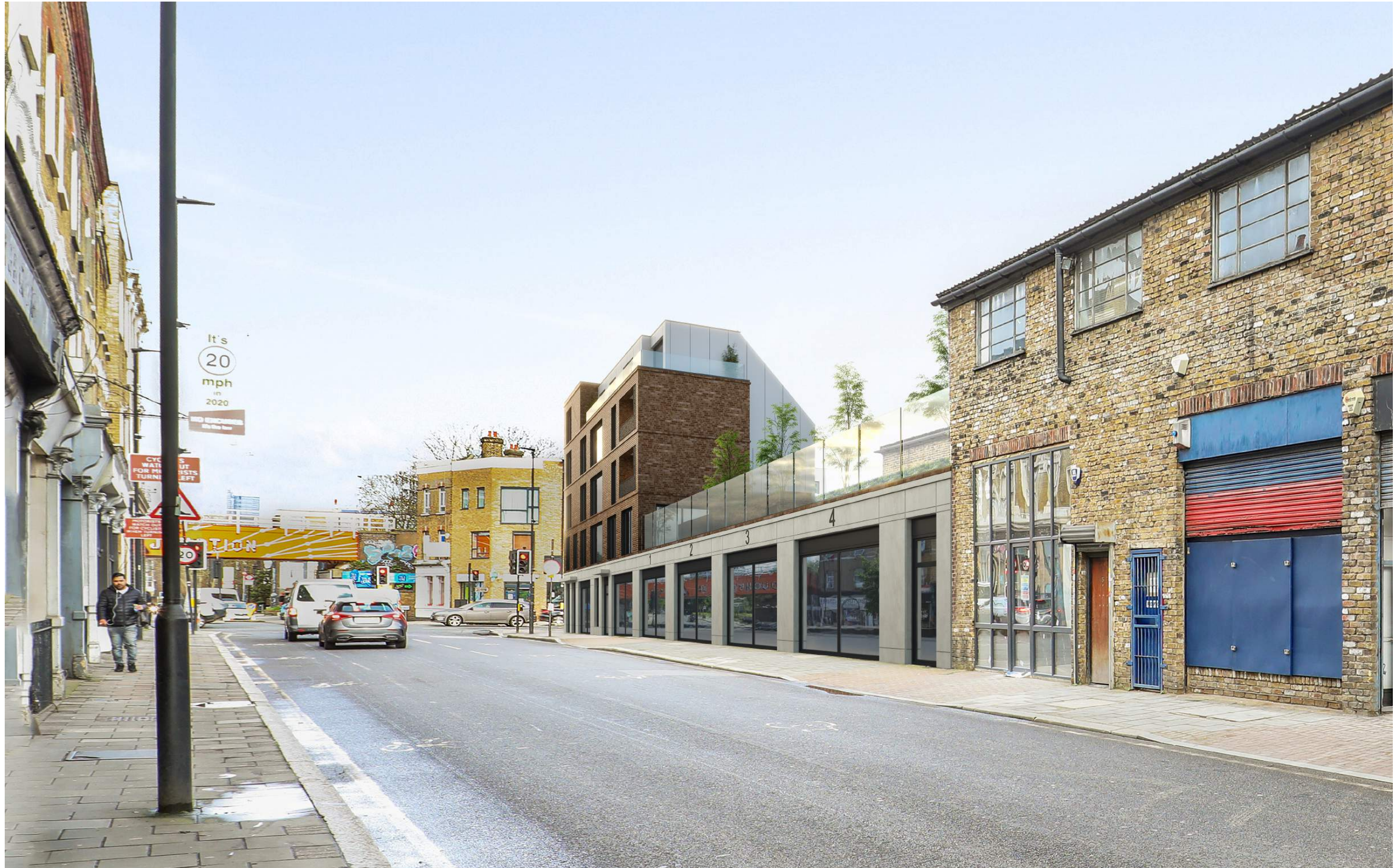
View NE along Coldharbour Lane
