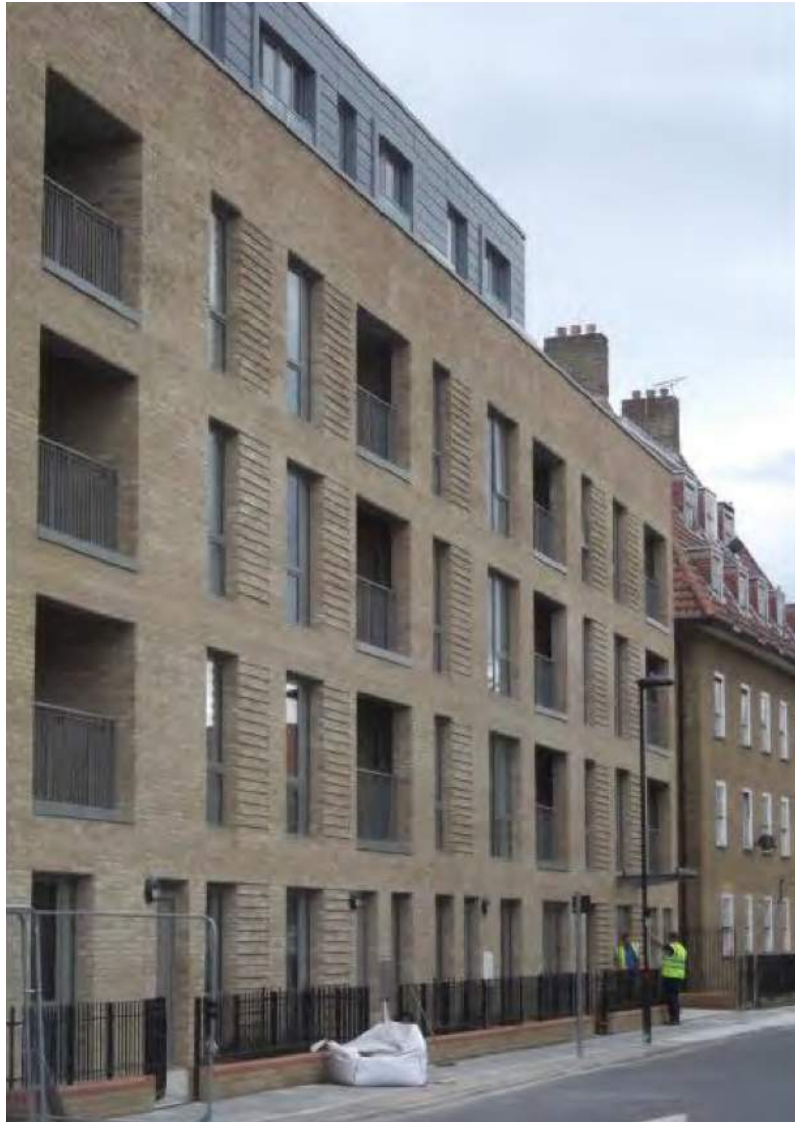
19. Sancroft Street showing brick facade and grey fenestration with recessed balconies and window openings, and grey clad penthouse level set back.
