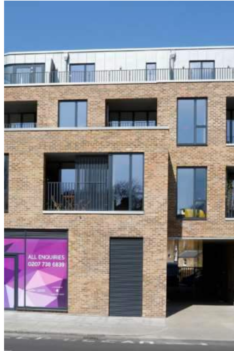
20. 207 Gipsy Hill showing layered brick elevations with varied rectangular openings and metal clad penthouse level
