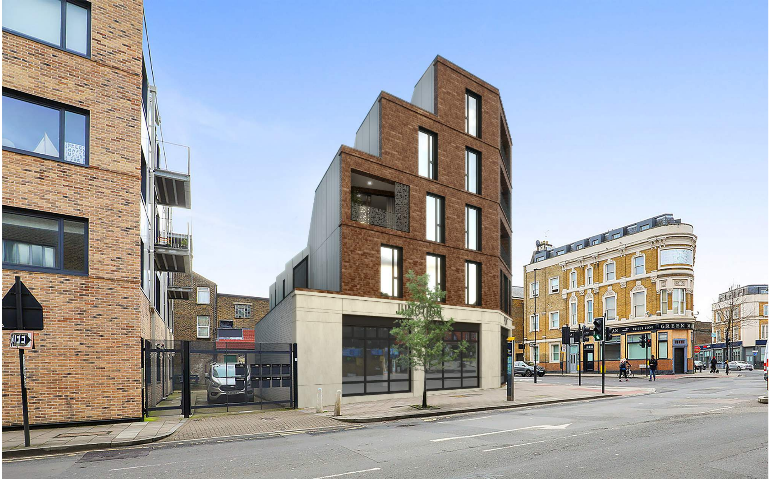
View SW along Coldharbour Lane
