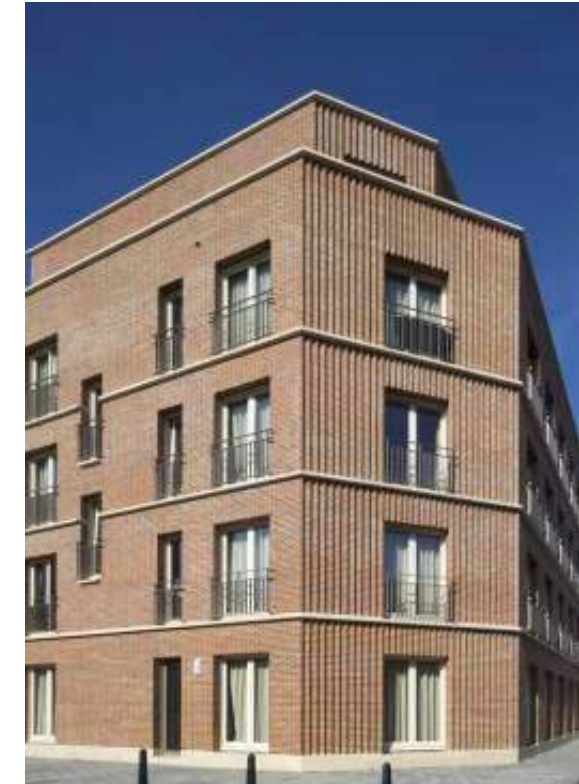
Example which has good profiling detail on brickwork to add interest to corner with well-integrated top floor setback
