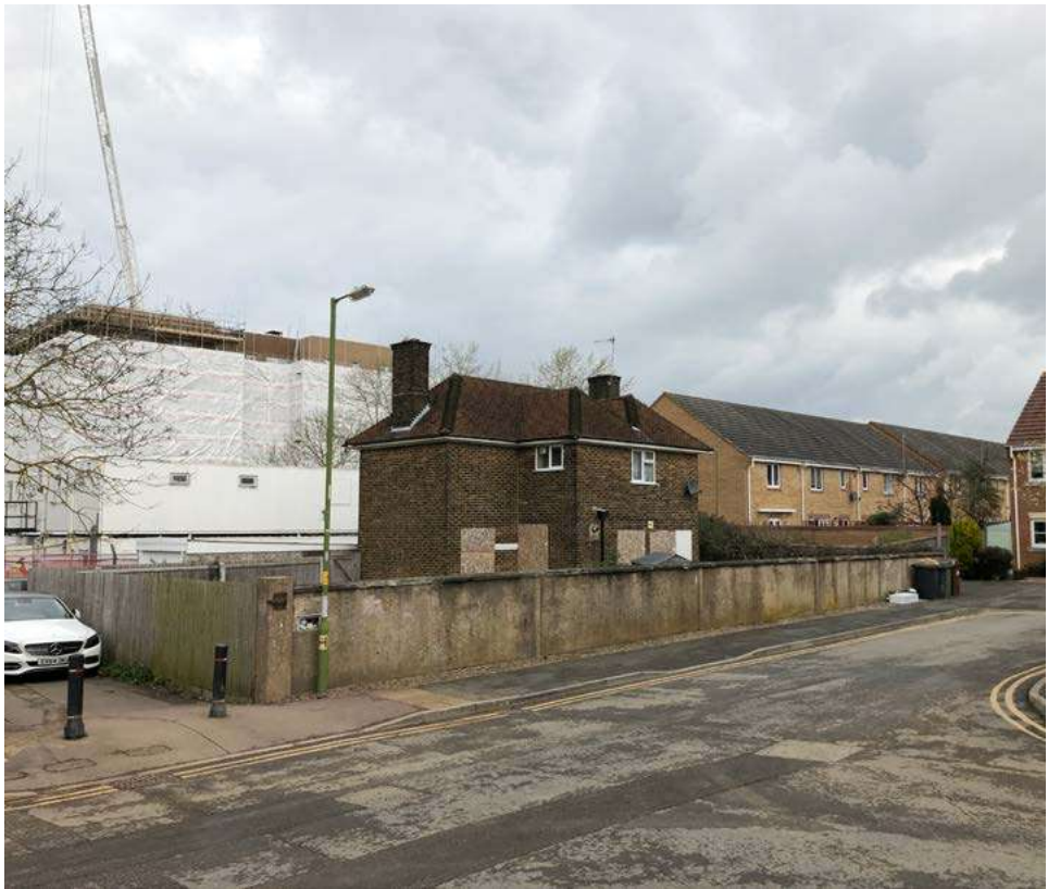
View of site from South West.
