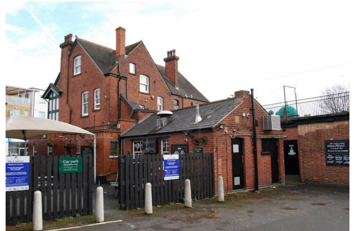
4 The site from the rear car park of The Goat looking South East
