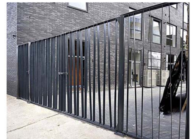
10 - Zig zag metal vehicular gates
