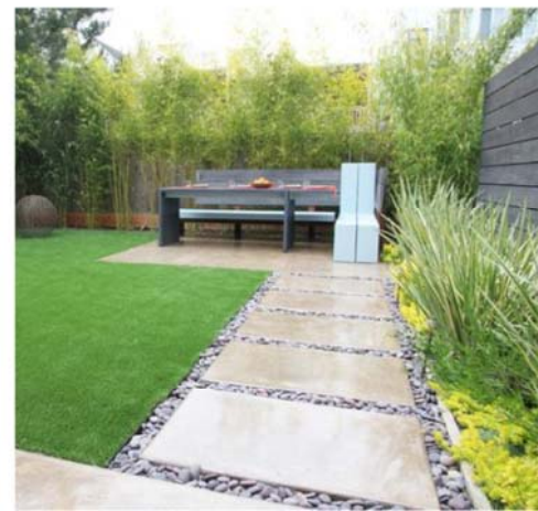
4 - Inset slab paving
