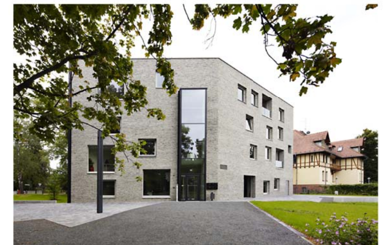
Example building with white brick
