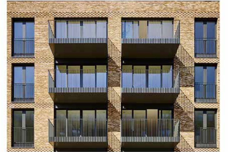
Balconies formed from metal flats
