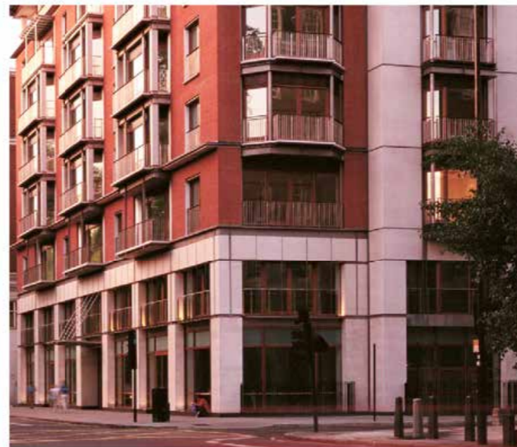
Stone cladding to ground and first floor elevation, squared off / angled bay windows and balconies in contrasting material
